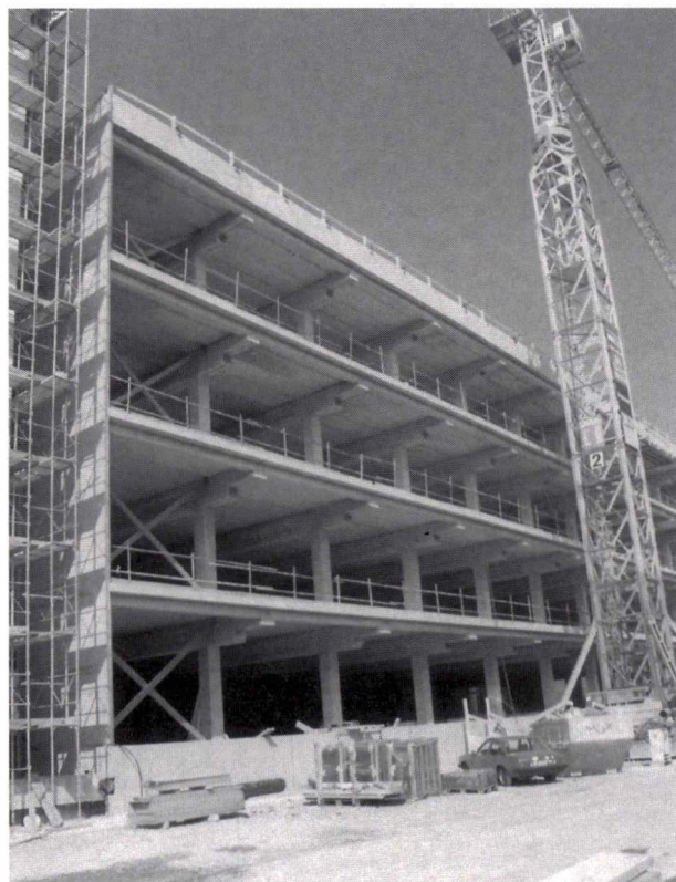
Bild 8: Foto Bauzustand Fig. 8: Photo operation building under construction
