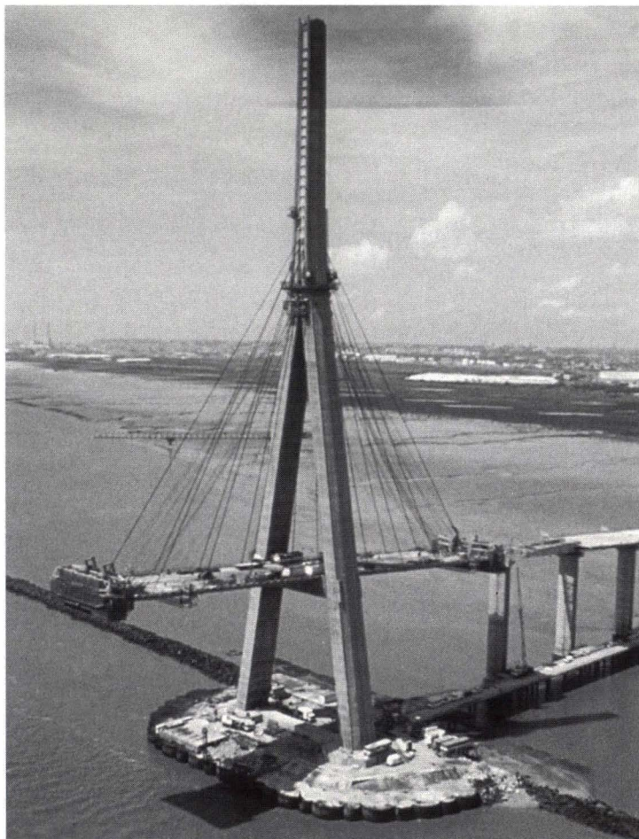
Fig. 6: Construction of the Normandy bridge (France)
