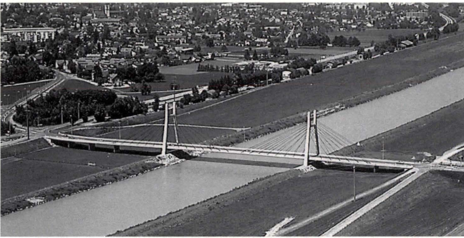
Fig. 9: Diepoldsau bridge (Switzerland)
