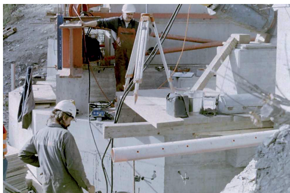
5 Spannen der Anker Tensioning of ground-anchor Tensioning of ground anchor
