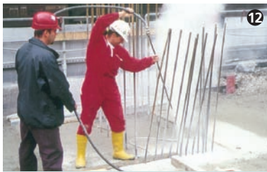
Bohrlochreinigung. Cleaning of the pre-drilled holes.
