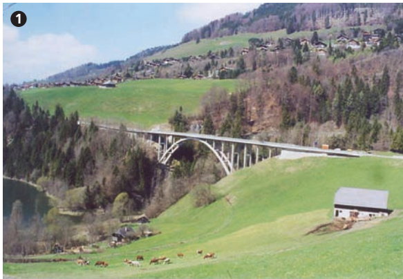
1 Situation du pont sur le Javroz. The Javroz bridge and its surroundings.
