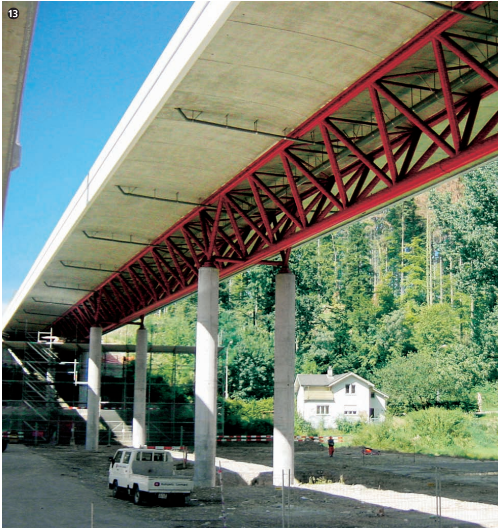
Die fertige Brücke. The completed bridge.
