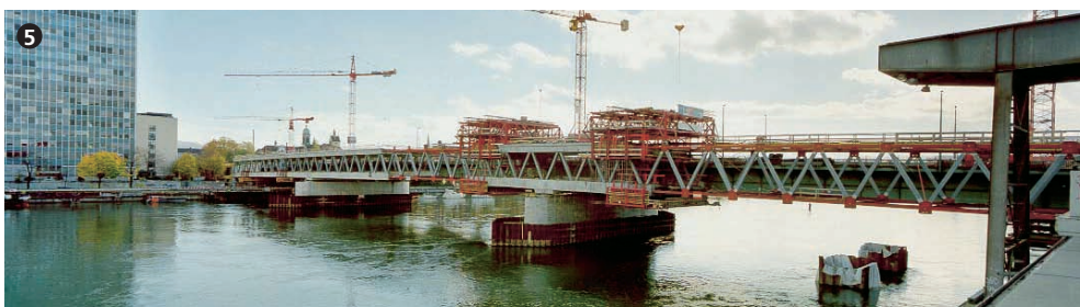
Nordbrücke im Bauzustand. North bridge during construction.
