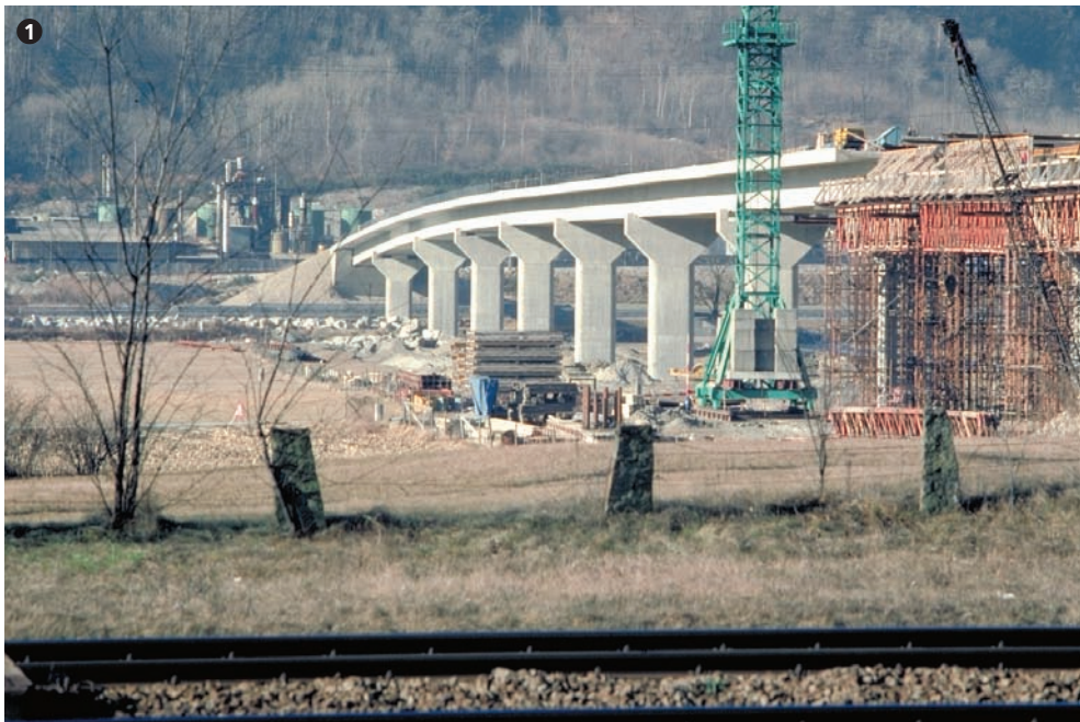
Ansicht der Brücke im Bauzustand. View of the bridge during construction.
